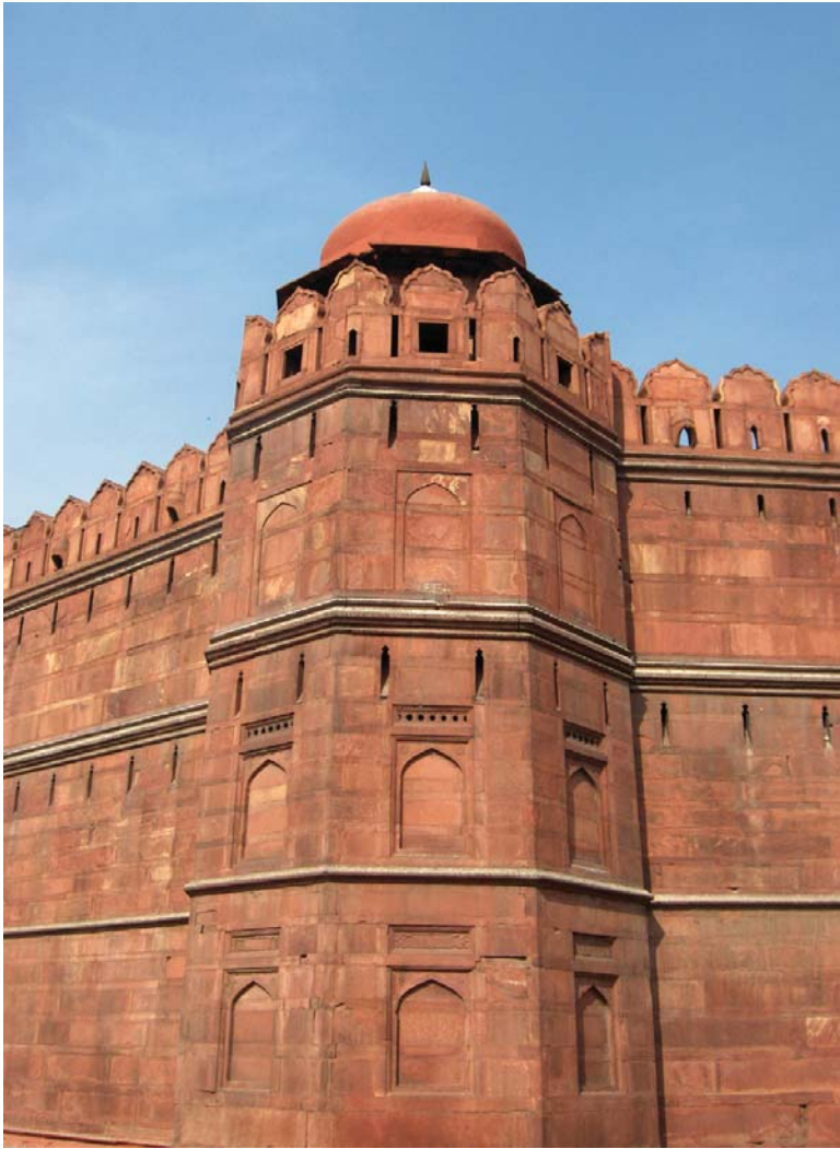
The sandstone of which the Red Fort in Delhi is built is a sedimentary rock.
